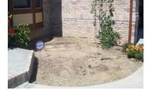
Dig a big hole, and create a perimeter of cement pavers. This creates the "pool" of water which will recycle into the fountain. I used 8" X 16" cement pavers. Secure the pavers by placing several inches in a trench and back-filling the trench. Use a level across the top in all directions.
