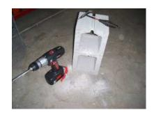
Determine the set-up of the pots for the fountain. Carefully located the cinderblock/s so the pot/s will be situated on them. Insure that it is level across the top of the cinderblocks and both sides of the pond. You may need to remove the carpet and pond liner to adjust the level.
