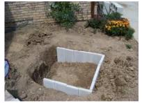
Line the pool with a layer of carpet (old, used or leftover) then cover with a layer of pond liner material.
