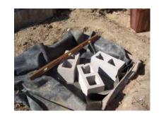
Tuck in the liner, nice and tidy, around the perimeter bricks. Run the pump tubing up through the cinderblocks using elbows and t's as needed. Dig a trench for the electric cord, use a PVC pipe in the trench and push the electric cord through the PVC. The electric cord should drop down into the pool at one of the corners.
