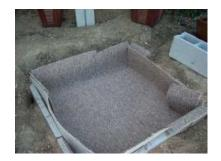
The cinderblocks may need to be modified to make room for the pump tubing which will run up through the cinderblock holes—a chisel or a drill with a masonry bit will do the trick.
